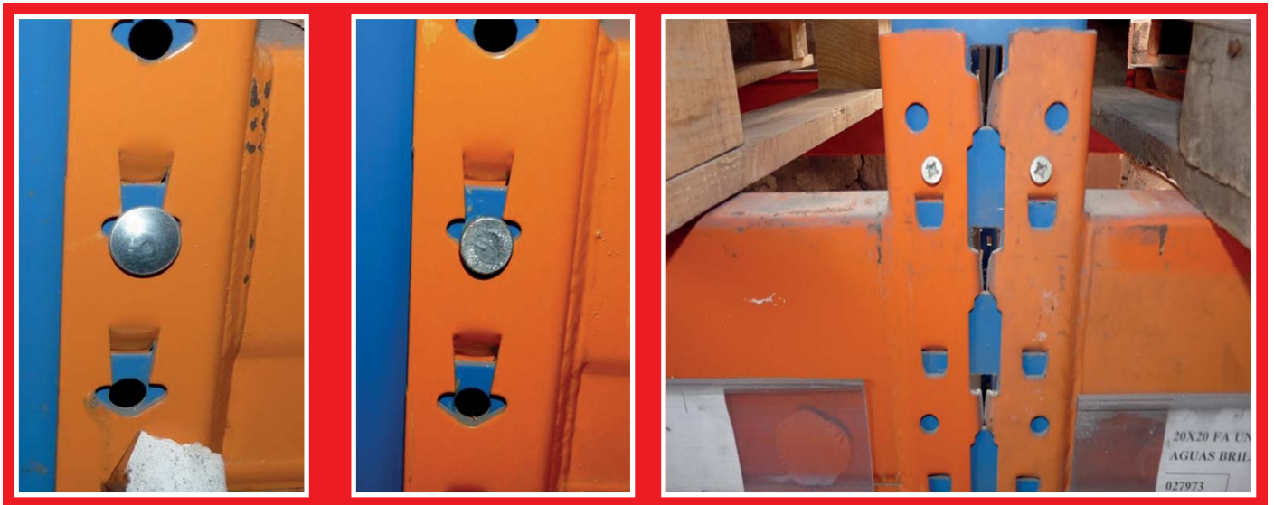
Securing Pins - wrong kind.
