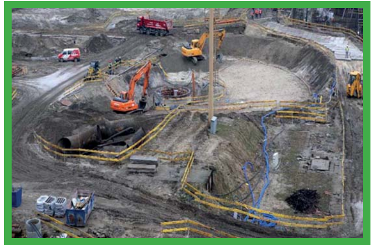
Transport systems at a construction site.
