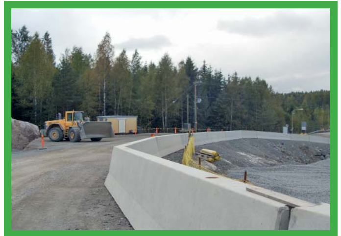
Edge Protection using precast structures.
