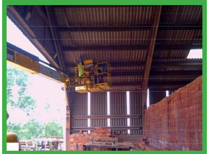
MEWP's in operation in brick manufacturing and cement production.
