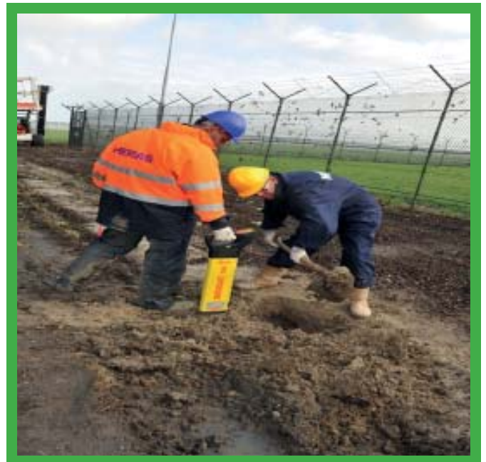
Checking for the presence of underground services prior to the erection of fencing.
