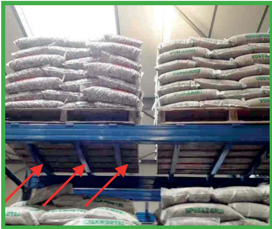
3 supporting beams for storage pallets.
