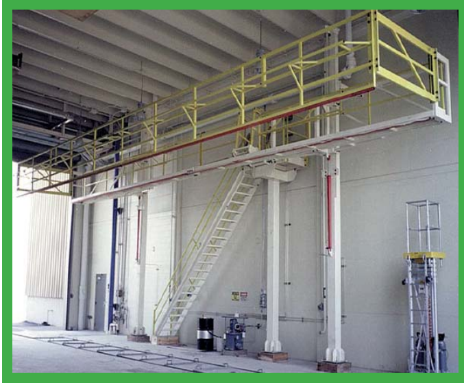
System at Finnsementti to protect the tanker driver during loading. This system has to be adjusted in terms of length and height to cover all vehicle sizes.
