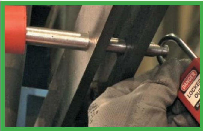
Mechanical Isolation: protecting a sliding door (Mechanical + Padlock).
