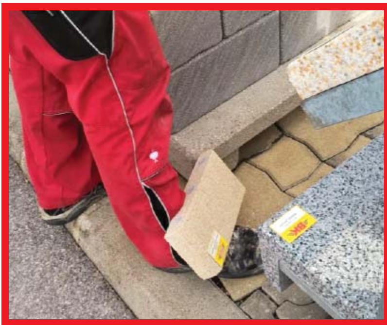
August 2017 accident: contractor suffered serious foot injury after blocks landed on area behind the steel toe cap shoe and struck the area that would have been covered by a metatarsal shoe or boot.
