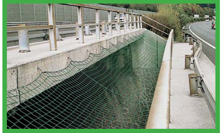
Safety Netting in place.
