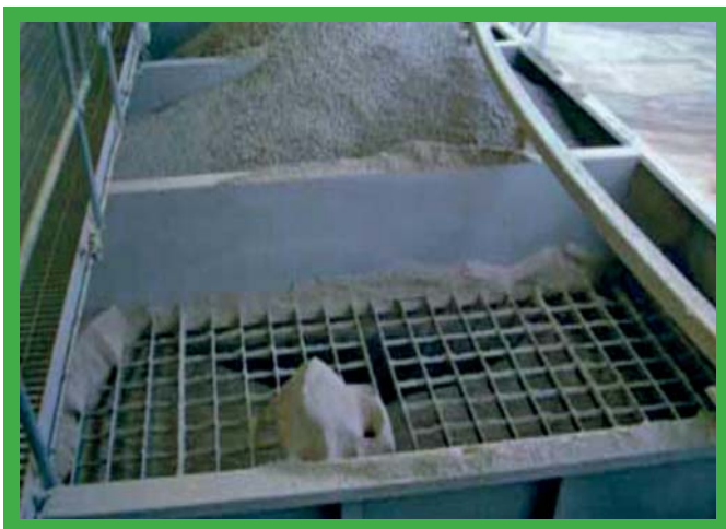
Man grids in place.
