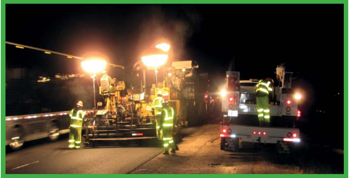
Road-surfacing at night close to live traffic.
