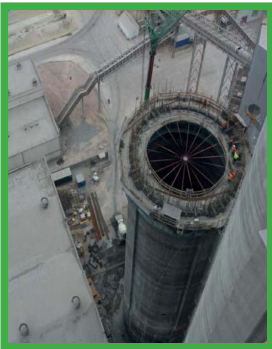
Raw Meal Silo Project.
