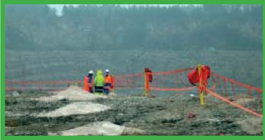
Barrier system at quarry face.
