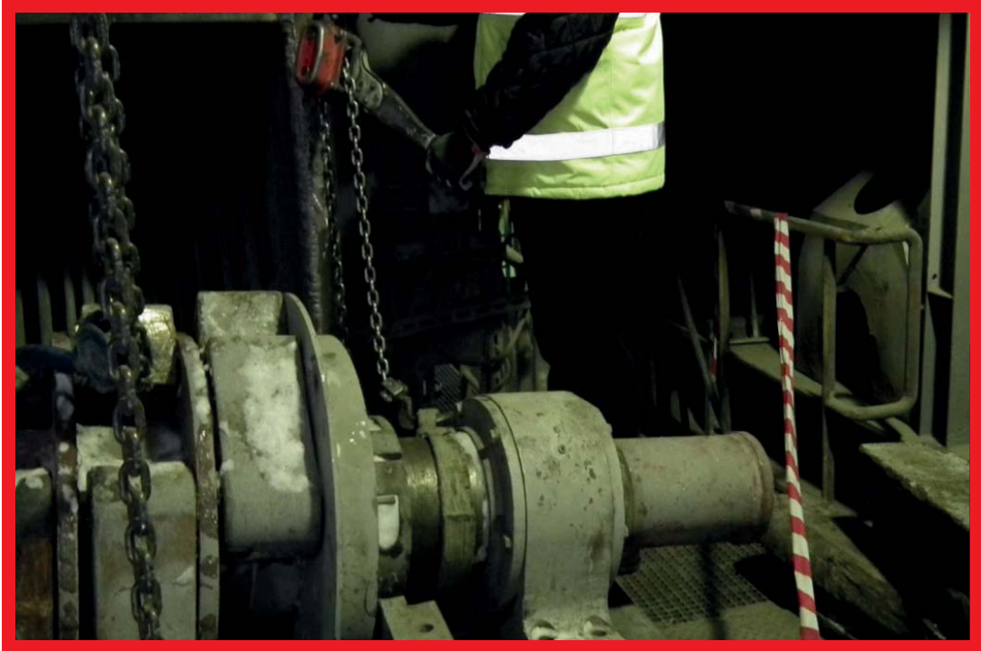
Serious Accident 2014: Accident involving major contractor firm: lifting gear failure during a lifting operation. Lifting gear certification out of date, task safe system of work incorrect.
