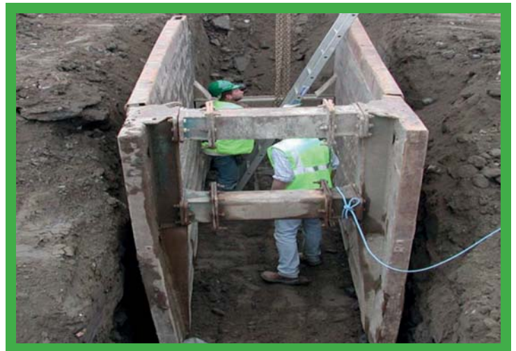
Trench Boxes in use.
